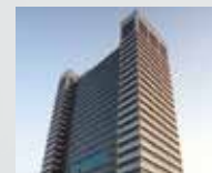
NIDEC DRIVE TECHNOLOGY TAIWAN CORPORATION (TAICHUNG, TAIWAN)
